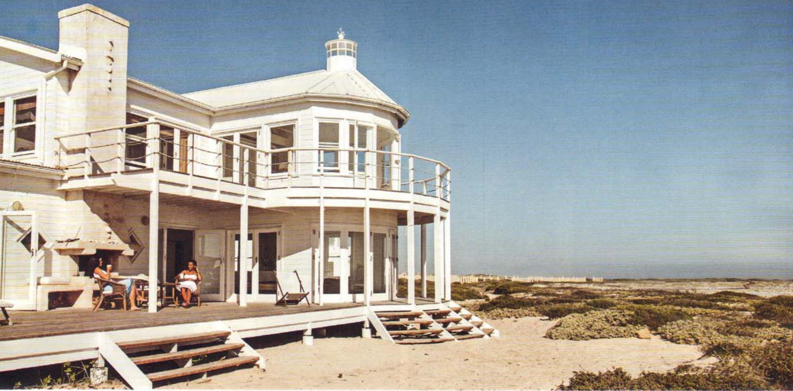
Clockwise from this picture: the open-plan sitting room and exterior of The Lighthouse; a path to the private beach in front of the property
